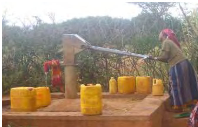
Figure 4.2: Protected hand pump well, Sirba village
